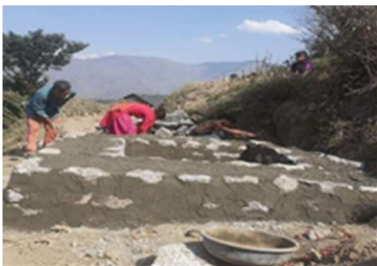
Irrigation tank being constructed in village Huded
